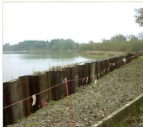
The sheet piling of the Warnham mill dam. Picture - Nigel Harris
